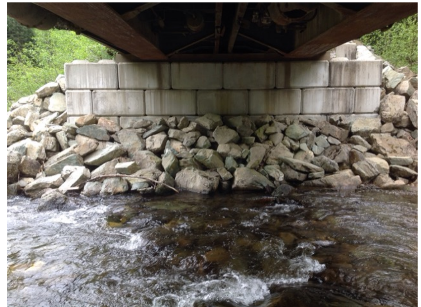
Right Bank Abutment when facing downstream
