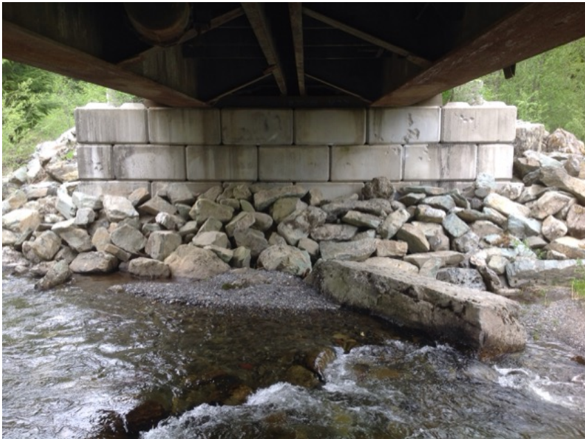
Left Bank Abutment when facing downstream
