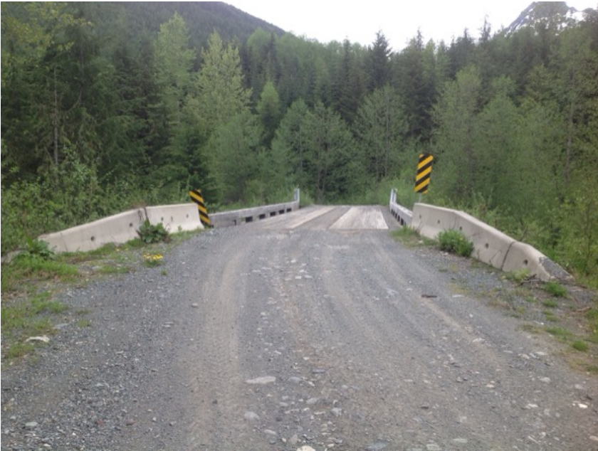
Approach from Right Bank when facing downstream
